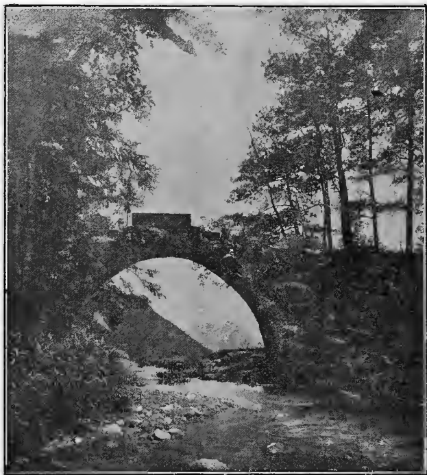
BRIDGE NEAR WUN-CHAU.
