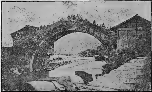
BRIDGE AT NING-KONG-GYIAO.
